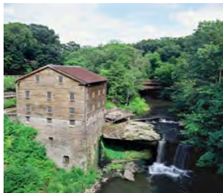
Mill Creek Metro Parks Lanterman's Mill
